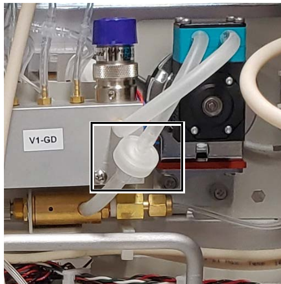
Figure 84: Replacing the Disc Filter
