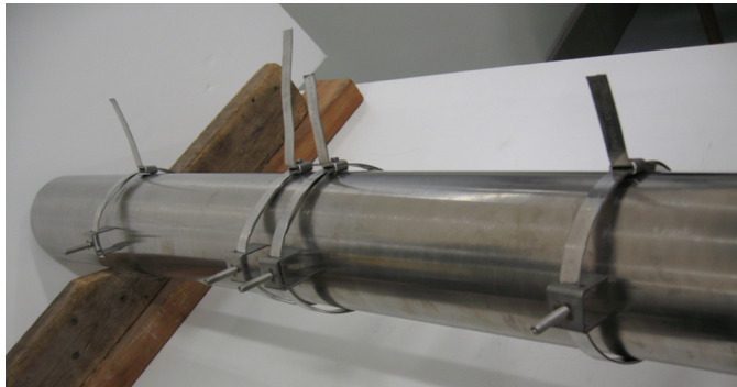
Figure B-31 Strap retainer and strap installation
