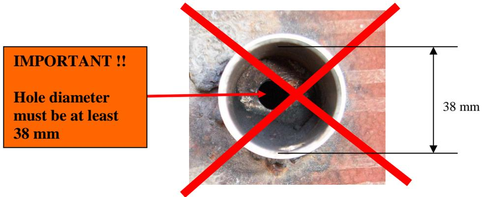
Figure 4. **Wrong socket installation,**
