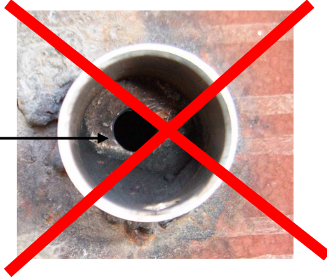
Figure 3b. Wrong socket installation, THE DIAMETER OF THE HOLE MUST BE MINIMUM 38 MM
